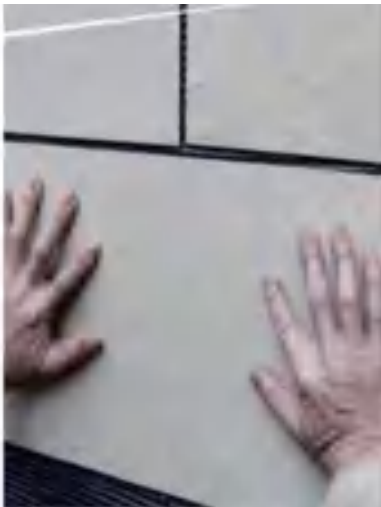
Adjust the width of the gap and pat it firmly
