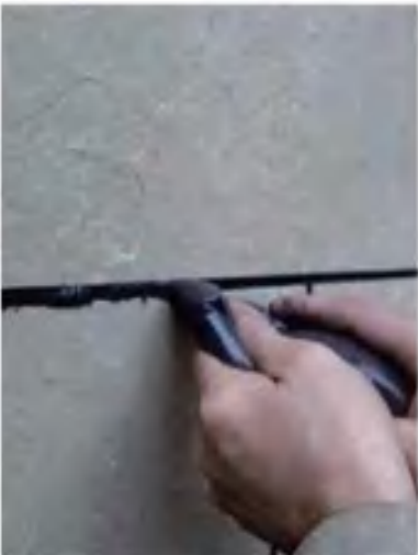
Grouting with grout
