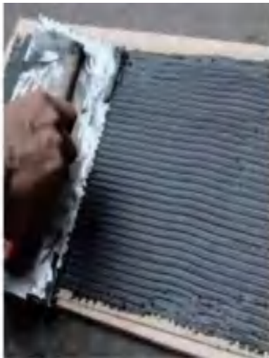
Apply Mortar To The Back Of The Product
