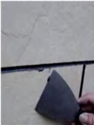
Remove the excess with a scraper
