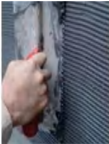
Apply Bonding Mortar To The Wall Surface
