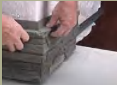
Corner approach : 45-degree splicing
